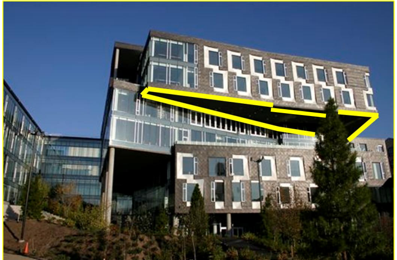
Image 23: Image of west façade with highlighted cantilever
